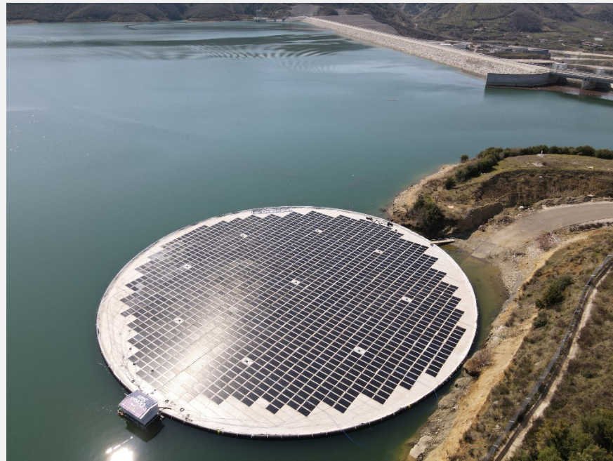
The first of four planned floaters for Statkraft on the Banja reservoir in Albania. The floater is ~3,700 m 2 and has an installed power of 0.5MWp.
